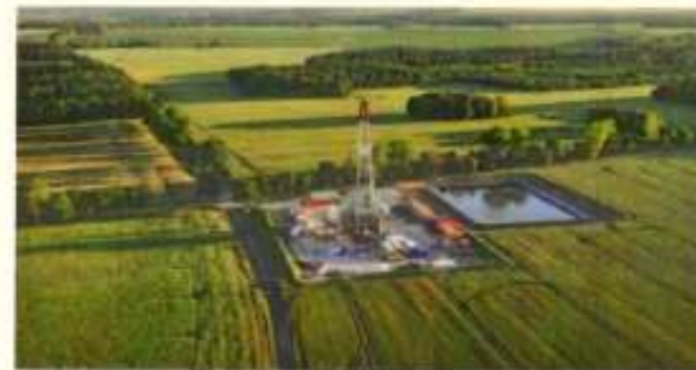
Pad during drilling (1 year)
