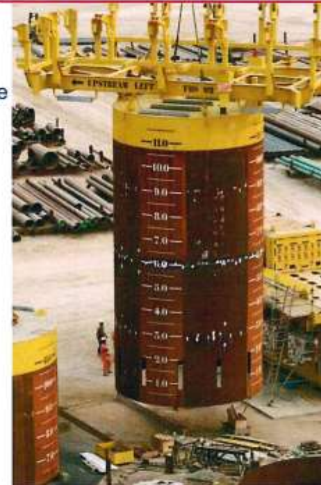
Foundation & Bottom Structure Leveling system (+/- 5°)
